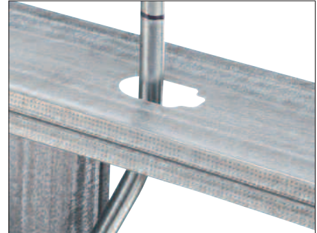
2 EMT marked and ready to cut.
